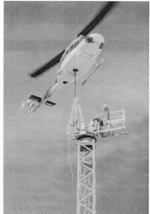
Helicopter cargo hook scales improve safety and productivity of field and air crews.
